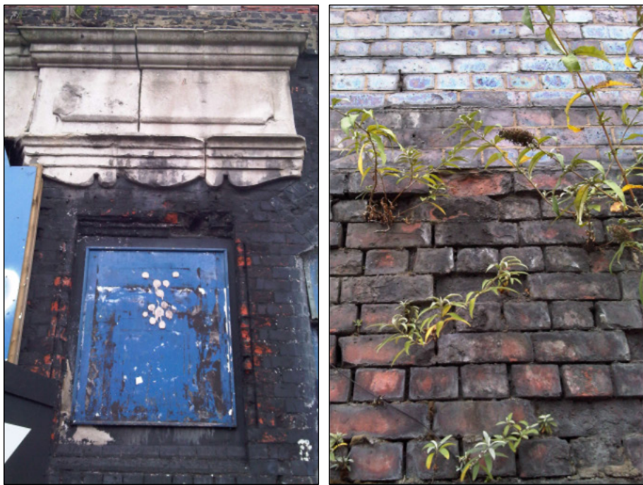
REPAIRS TO BRICKWORK & ORIEL STRUCTURE - This work will include vegetation removal, repointing and replacement of badly spalled or missing bricks.
